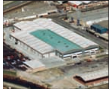
Product premises of Cooper Crouse-Hinds (UK) Ltd., location Sheerness, UK
