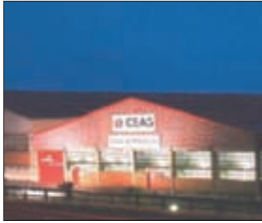
Production premises of Cooper Crouse-Hinds S.A. location Terrassa, Spain
