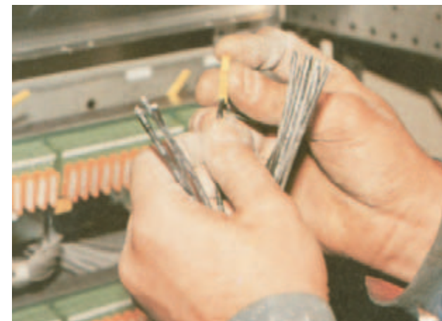
COMPUTERIZED MULTI-CHARACTER MARKING MEANS THAT ALL MARKING INFORMATION IS PRINTED ON A SINGLE SLEEVE WHICH CAN THEN BE SLID INTO PLACE VERY EASILY AND QUICKLY.
