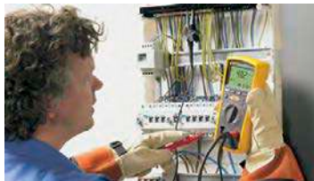
Insulation test at a distribution panel
