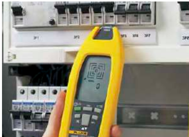
Location of fuses/breakers and assignment to circuits
