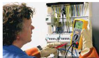
Insulation test at a distribution panel
