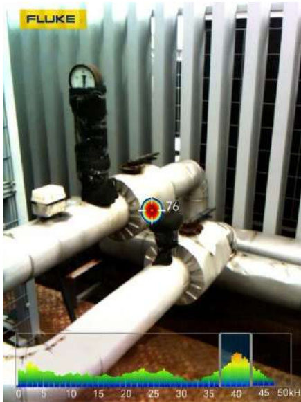
Leak detection on a pipeline
