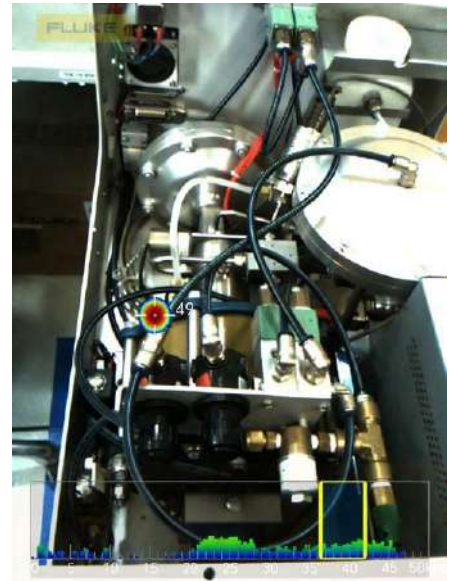
Air tightness inspection of complicated equipment pipelines
